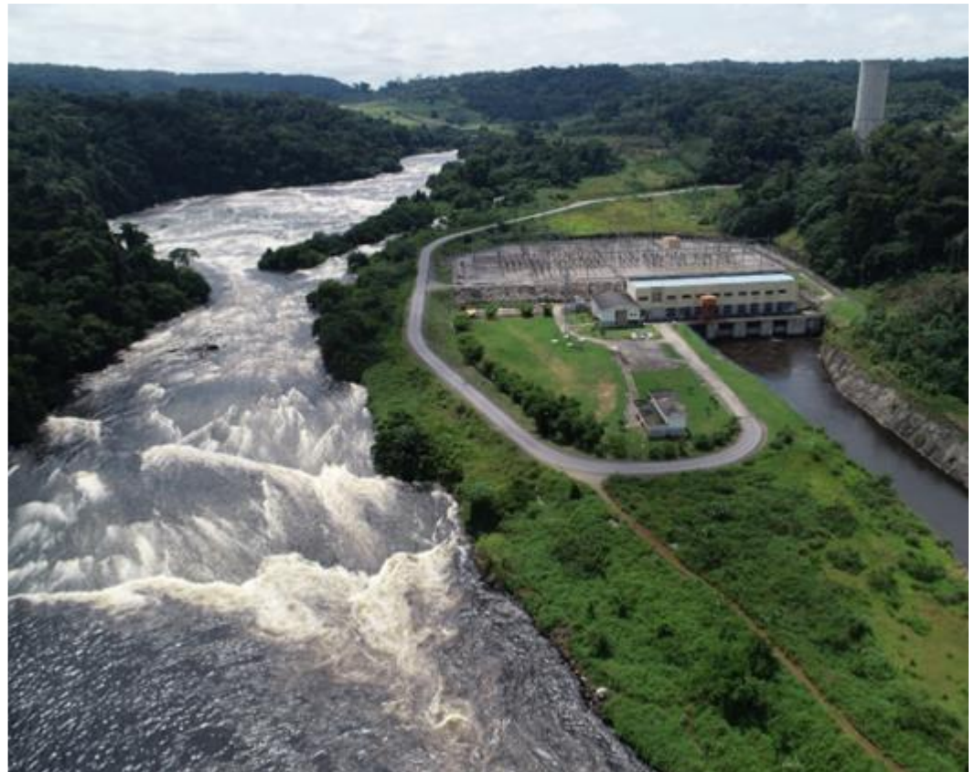
Figure 4: Grand Poubara Hydroelectric Power Station
