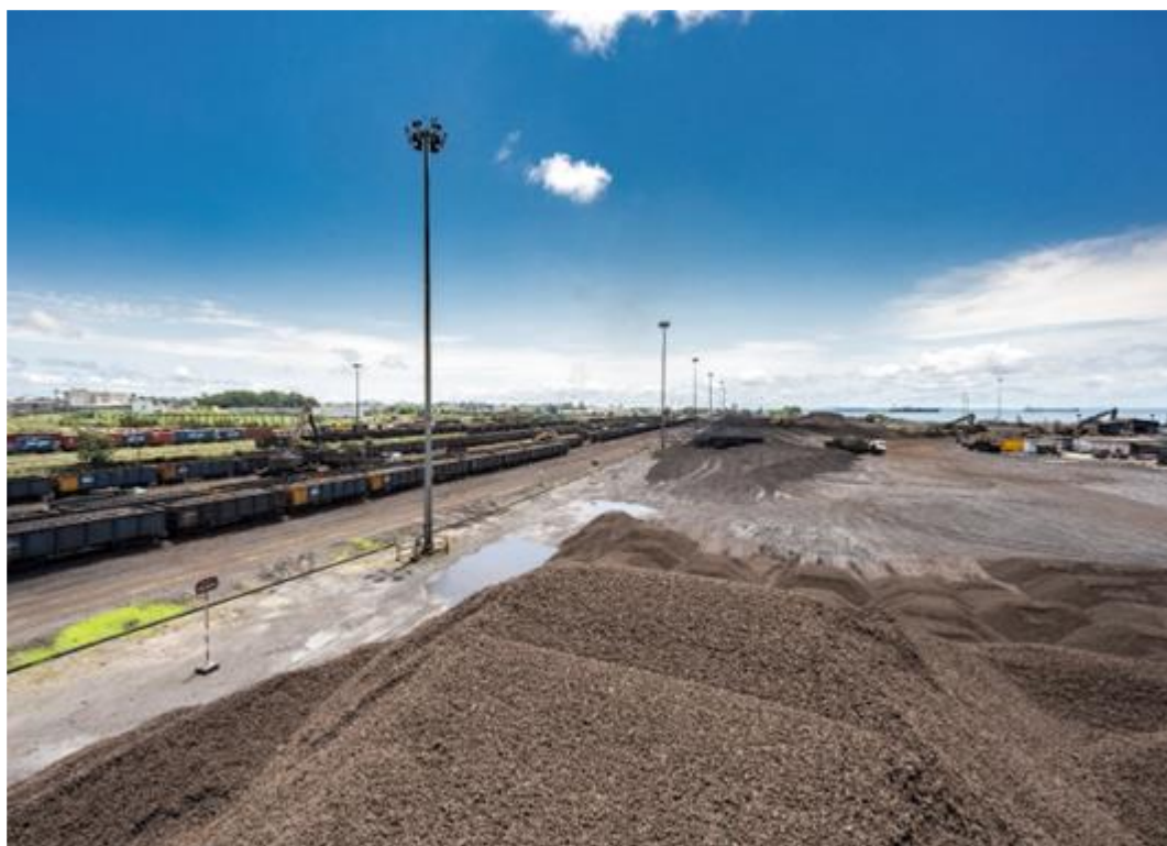
Figure 3: Rail and port facilities at the Owendo Mineral Port
