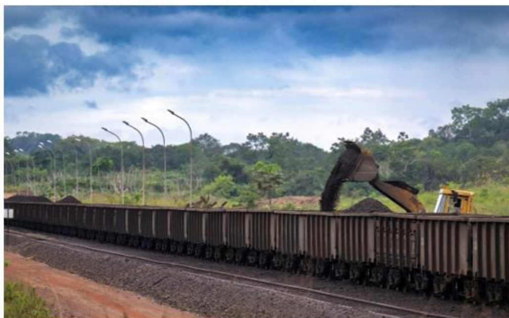
Figure 2: Rail and port facilities at the Owendo Mineral Port near Libreville
